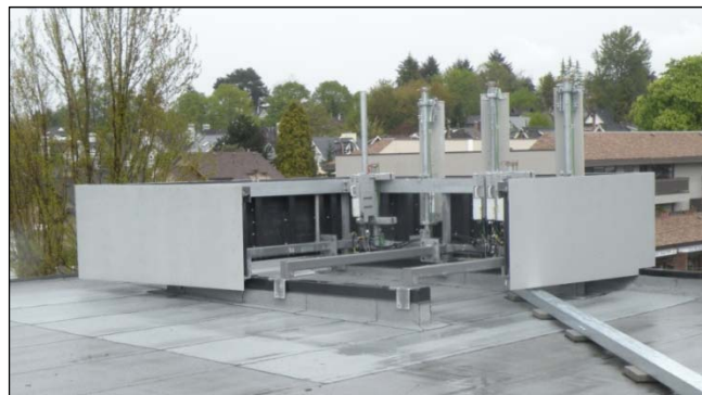
FRP Panels and structural materials were used to build a shroud around the cellular antennas.
